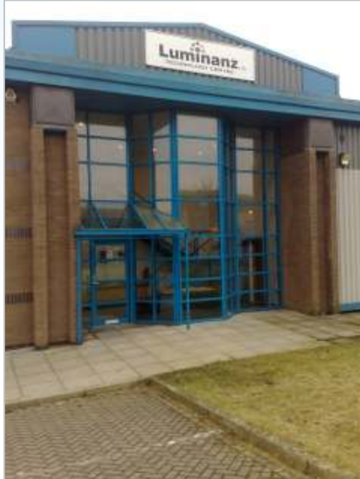
Luminanz Ltd Bolton, UK
